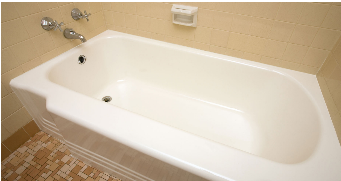
Figure 2: Modern private bathtub [3]. Facuet and overflow drain are in the left end of the bathtub.
